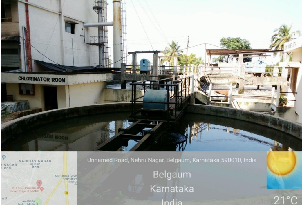
Sewage treatment plant
